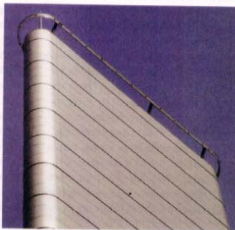
The fall arrest system was designed to fit the appearance of the stack.
